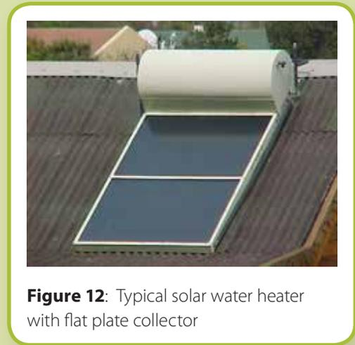
**Figure 12:** Typical solar water heater with flat plate collector
