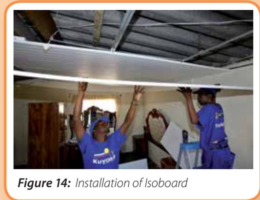
Figure 14: Installation of Isoboard
