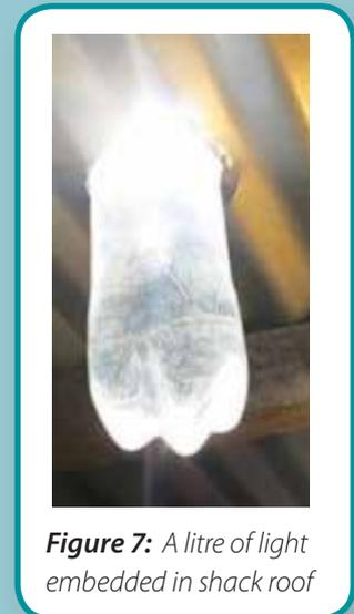
**Figure 7:** A litre of light embedded in shack roof
