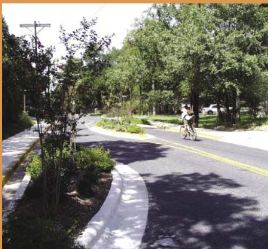
Chicane planters in suburban street, to slow down vehicles and encourage non-motorised transport (Source: City of Austin)
