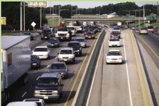
HOV lane is designated by the diamond symbol. This lane can only be used by cars with 2 or more passengers (Source: Dallas Area Rapid Transit)
