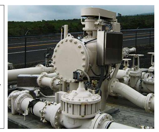
Water entering a reservoir still has excess energy that is normally dissipated by means of pressure control/reducing valves (PRVs) to avoid damage to pipe inlets. A parallel dissipating system, a water turbine, can be installed.
